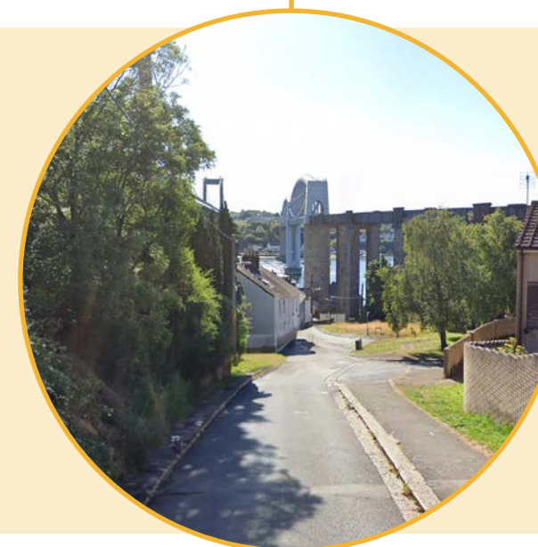
Picture of the Royal Albert Bridge from Lower Fore Street in 2023.
