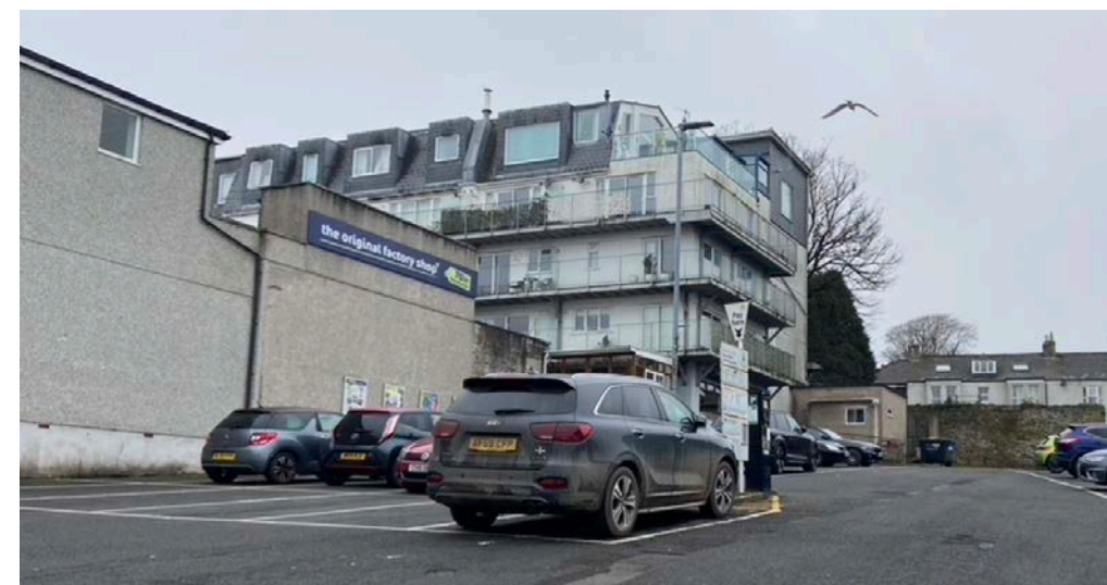
Belle Vue Carpark West
