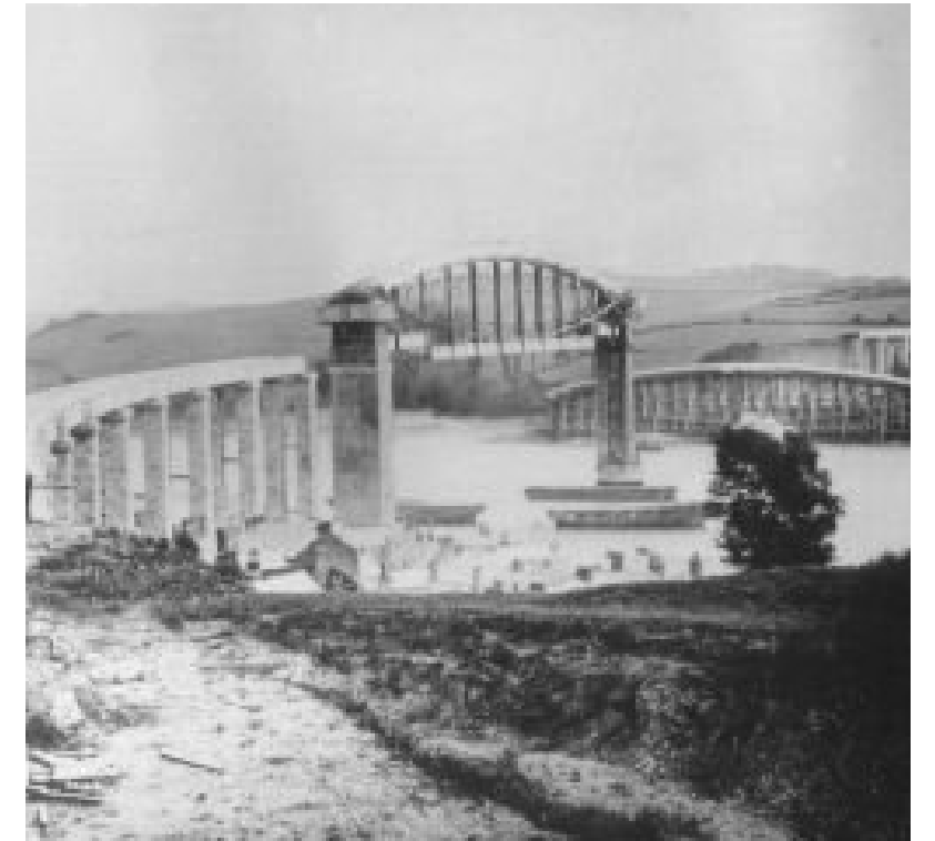
The Prince Albert Bridge construction in 1857 before opening in 1859
