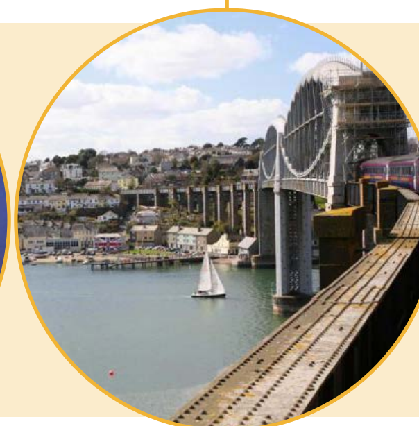
Picture of the Royal Albert Bridge in today from the eastern end.
